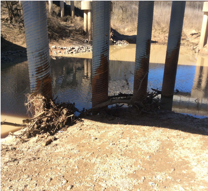
PHOTO 1 Description Bent 4 Piles 1-4 (no debris build-up)
