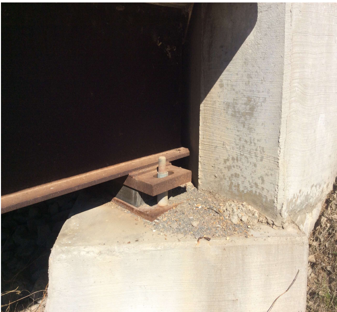
PHOTO 1 Description Bent 6 Bearing 5 right (nut missing)
